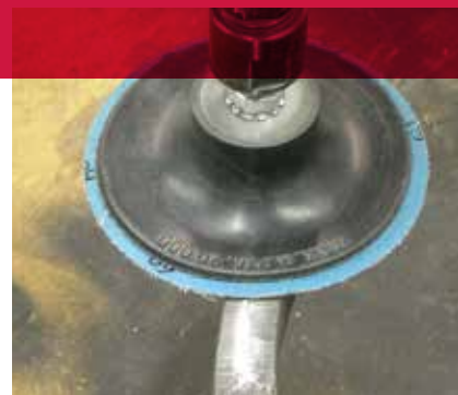
Blending surface imperfections prior to painting.
