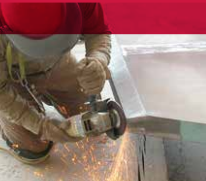
Grinding on a platform for weld preparation.
