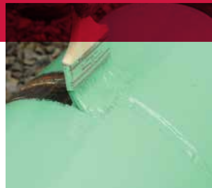
Applying pipe coating to weld seams.
