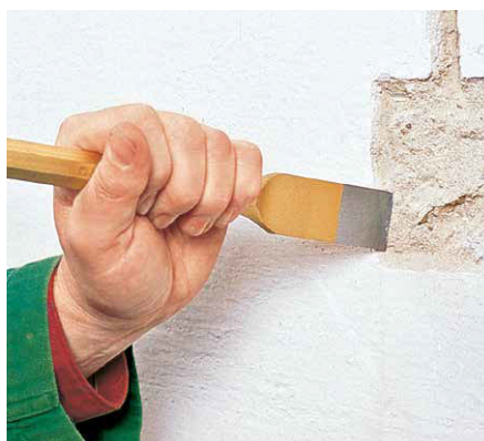
Schlitzmeißel, 8-kant Slotting chisels, octagonal
